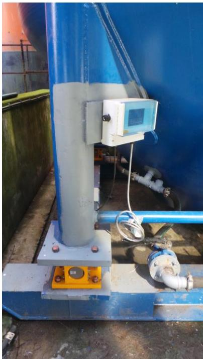
Euroload Limited manufacture a purpose built display for silo content weighing.
